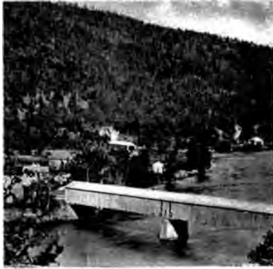
CONNECTICUT RIVER BRIDGE
